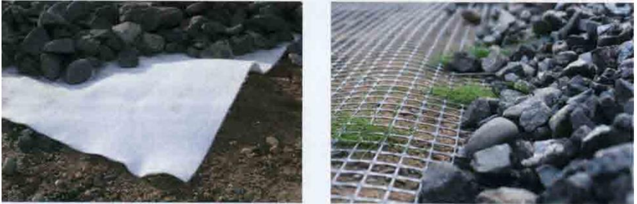
Fig. 2. Laying geotextiles and geogrid
