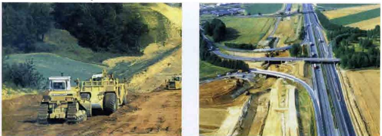
Fig. 1. Construction of the earthwork of high-speed railways
