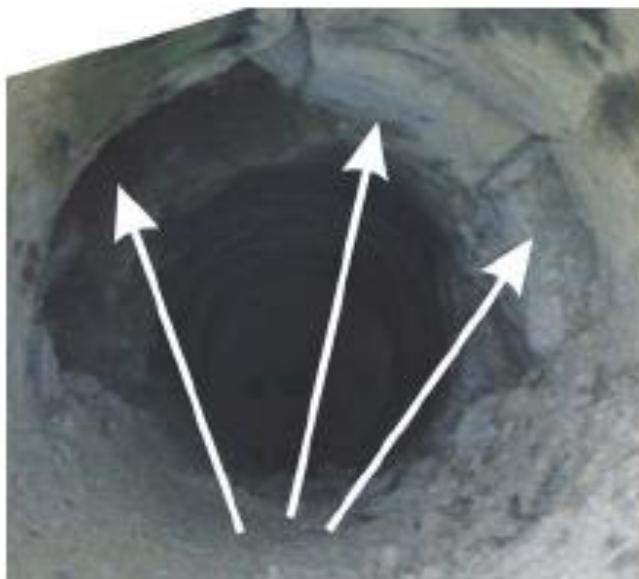
Fig. 3. The arrows mark the destruction zones of the external masonry (lining) of the pipe.
